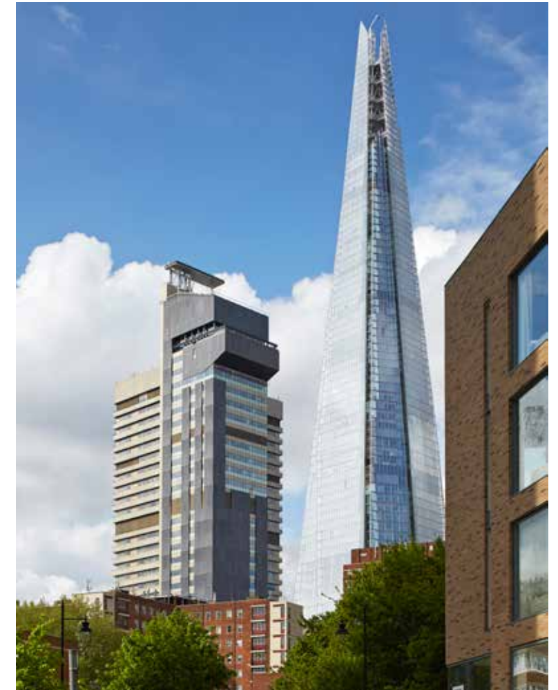
Image 8 Guy's Hospital overcladding designed by Penoyre & Prasad and the Shard, designed by Renzo Piano Building Workshop: have durable but distinct finishes on their aluminium building envelopes – anodising with an 80-year guarantee and Class 2 polyester powder coating with a 40-year guarantee, respectively
