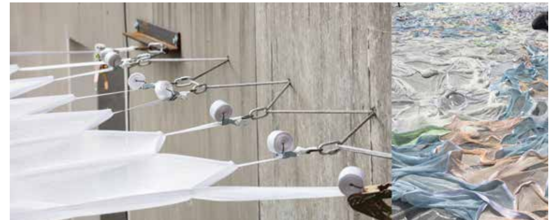
Images 25 & 26 Perimeter edge details and unfolding and preparing the canopy for installation; solar active yarns revealing their colors in the presence of the sun.
