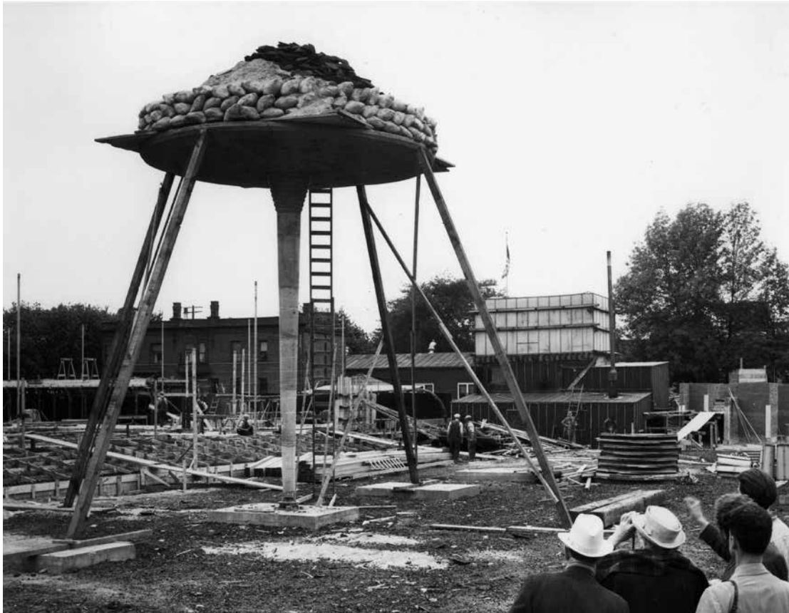
Image 15 Frank Lloyd Wright witnessing the testing of a prototype cast concrete column for the Johnson Wax Administration Building
