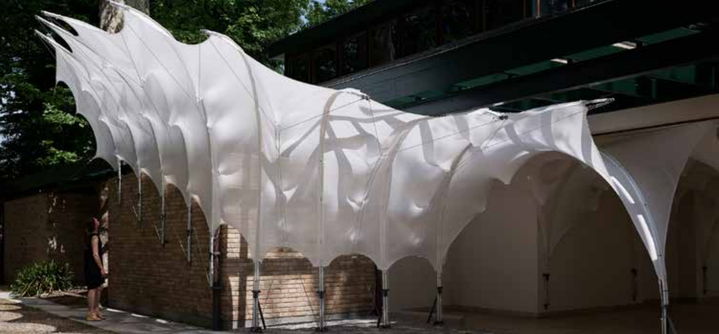
Image 5 In Isoropia , highly interdependent system of active bent GFRP rods and tensile membranes interact to create overall structural performance. These interactions are simulated employing projection-based methods (K2Eng) and correlated to Isogeometric Analysis (Kiwi). Martin Tamke, Mette Ramsgaard Thomsen, Yuliya Sinke in collaboration with AFF Filhos and Structure.
