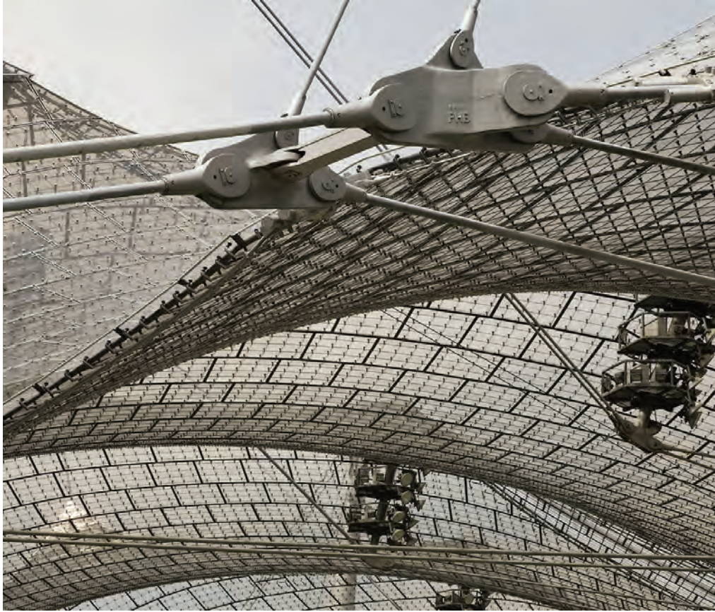
(4) Tensile roof detail, Munich Olympic Stadium, 1972
